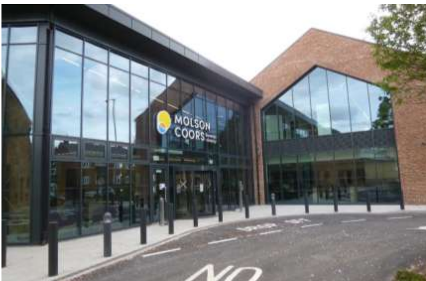
Top - the ornate ceiling in Old Bass House, the prospective site for the new centre. The 1866 water tower will form part of a larger visitor facility. Bottom - the new Molson Coors offices on the old NBC site.
