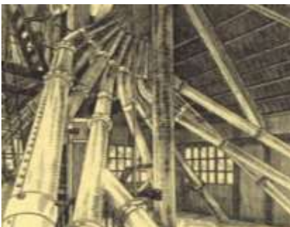
From Barnard's visit to Chiswell Street around 1890; the 14 tubes feeding the 1000 quarter malt bins, the porter tun room with its pontons and the cooperage yard. Strangely Barnard included just these three drawings in his piece about Whitbread.
