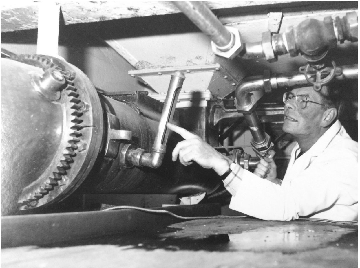
Figure 19. Mash tun Steels masher with head brewer c.1955.
