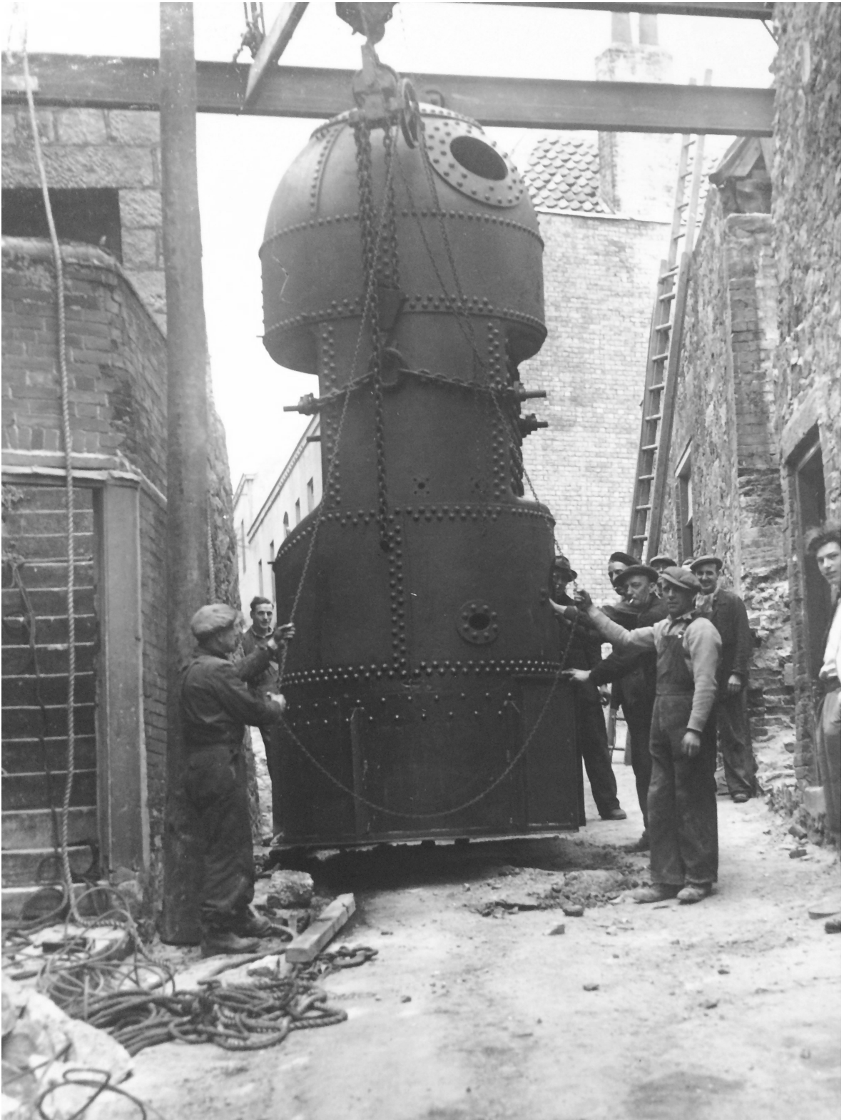
Figure 11. Boiler in final position pre second world war.
