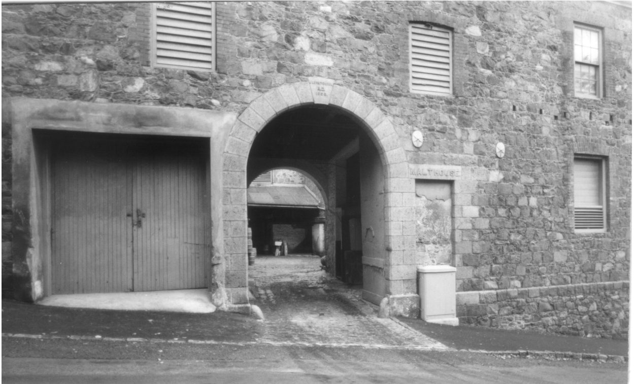
Figure 21. Malthouse entrance at side of brewery, Havelet Street, 1974.
