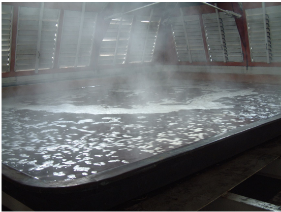
Figure 60. The open wort cooler at Hook Norton (2002).
