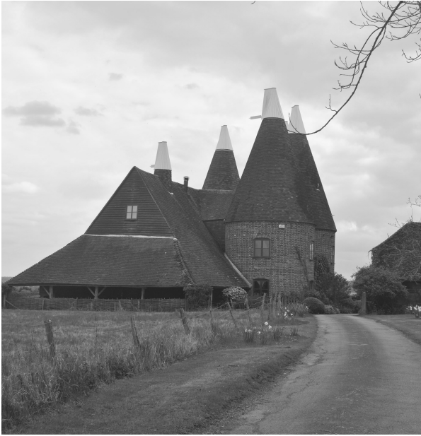
Figure 32. Many oast houses have been converted into houses; this one is at Chiddingstone in Kent.
