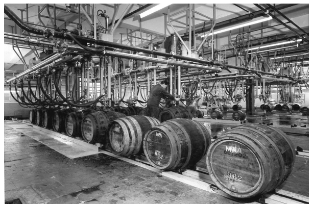
Figure 83. The racking room at Cape Hill, note the white-wash stencilled code. (NBHT).
