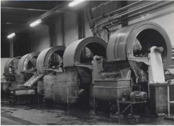
Figure 9. Rotary vacuum filters for drying yeast at Guinness in Dublin. Photo courtesy of Diageo Archive.
