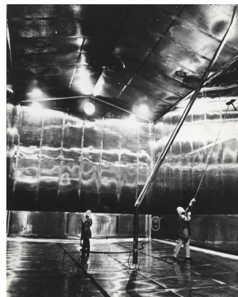
Figure 14. Scouring inside the 12000hL 26M fermenter at Guinness in Dublin. Photo courtesy of the Diageo Archive.
