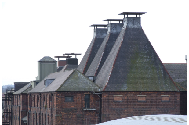
Figure 26. The kiln exteriors at W & D Langley Maltings.
