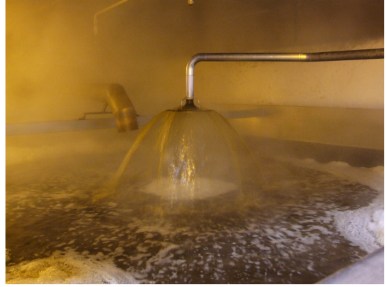
Figure 59. Casting over late hops at Theakston (2009).
