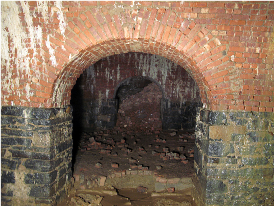
Figure 21. Vault 2: Doorway in the north wall to vault 3 with circular drain in the threshold, view of blocked doorway in the north wall of vault 4. Photo by Celia J. Bergoffen.
