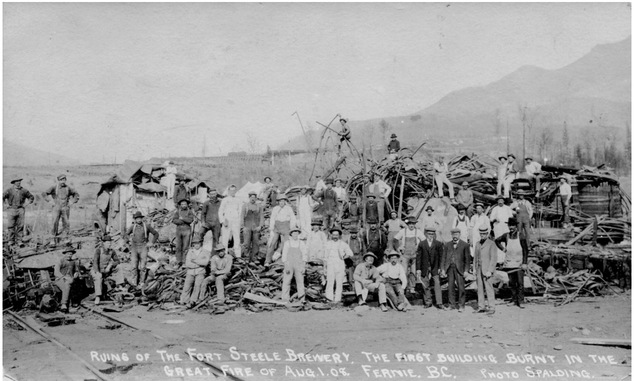
Figure 9. Mutz and a work crew prepare to clear the debris, August 1908. (Fernie Museum and Archives 1358).
