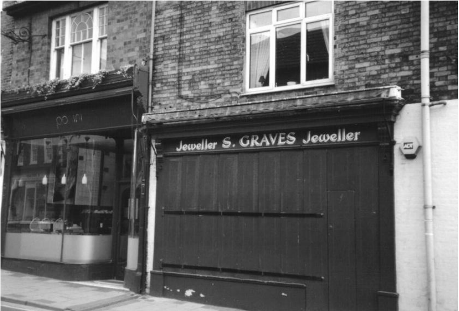
Figure 5. Shop fronts in Grantham showing increase in height and area devoted to windows (author).
