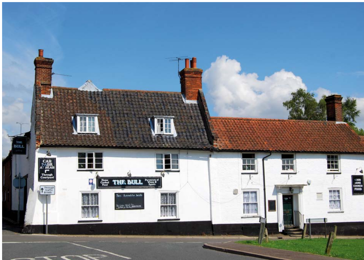
Figure 7. The Bull, Litcham, in central Norfolk: William Hardy's excise office 1768–69. Here he left the service when facing a third dismissal. Photograph Margaret Bird 2011.
