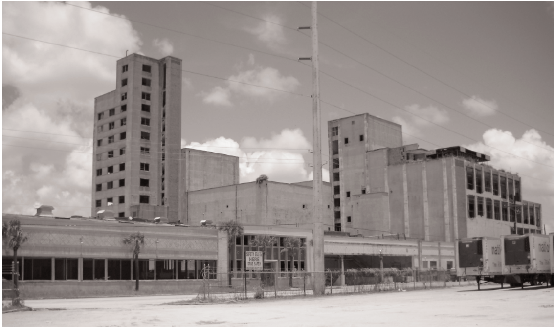
Figure 6. The south façade of the Falstaff Brewery photographed in June 2016. After the brewery's closure in 1981, the complex sat in a blighted state until rehabilitation projects began in 2016. (Preservation Resource Center; Galveston Historical Foundation, Galveston, Texas).
