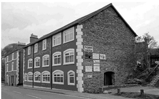
Figure 3. Sun Brewery malt-house. Photo: G.W. Stone, 2012.
