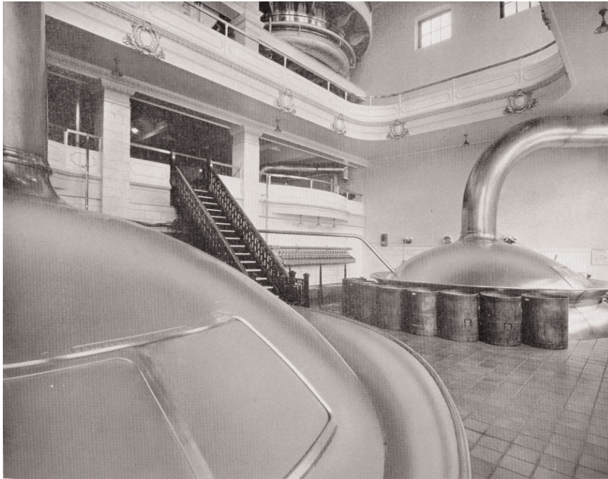
Figure 26. In 1911 Wolf completed a new brew house and power house for Philadelphia's Schmidt brewery. The brewing floor contained two 750-barrel kettles. This replaced the brew house he designed for Schmidt in 1887. This was the last of 33 projects that he did for this brewery. Anon (c.1940) C. Schmidt & Sons Brewing Co. Illustrated. Philadelphia, n.p.
