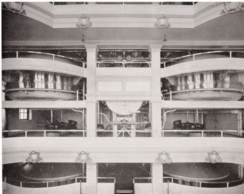
Figure 27. View of the lauter tubs overlooking the kettle floor below. Anon (c.1940) C. Schmidt & Sons Brewing Co. Illustrated. Philadelphia, n.p.
