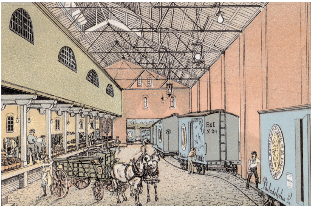
Figure 5. In 1886 Wolf made alterations to Bergner & Engel's ice house so wagons and cars could be loaded in a refrigerated environment during the summer months. (c.1888) Bergner & Engel Illustrated. n.p.
