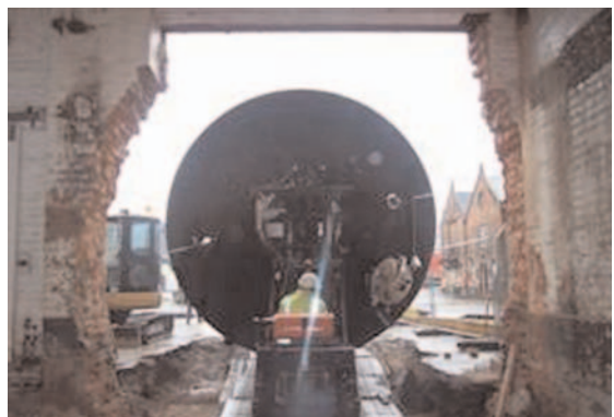
Figure 32. Marston's brewhouse expansion project 2004-05 (clockwise from top-left): original floors removed; creating the north elevation breach in bay 4; manoeuvring a mash tun section through the breach; moving a complete copper through the ground floor breach in bay 1; reconstructed ground-floor breach after completion; new operational brewhouse showing the three coppers at first-floor level, mash tun with grist hopper above to left and the girdled cast-iron columns (all photographs Copyright © Marstons plc).
