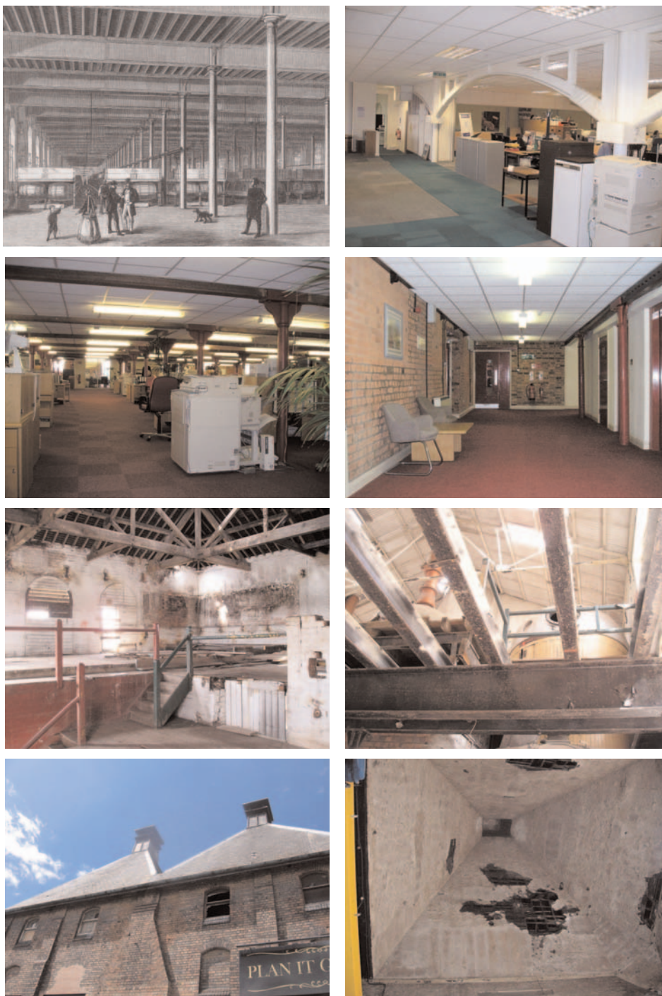
Figure 24. Highlighting some of the challenges of brewery building regeneration (from top); cast-iron column spacing dictates floor plans and headroom at the former Allsopp New Brewer tannery; deep plan forms limit cross ventilation and natural lighting levels inside former Bass malthouse No.20 at Wetmore; irregular storey heights, complex roof structures and fragile sheet roof coverings at the Everard Trent Brewery c.2005; falling plasterwork inside one of the kiln houses at Walsitch Maltings (archive image from Illustrated London News 1867; author's collection).
