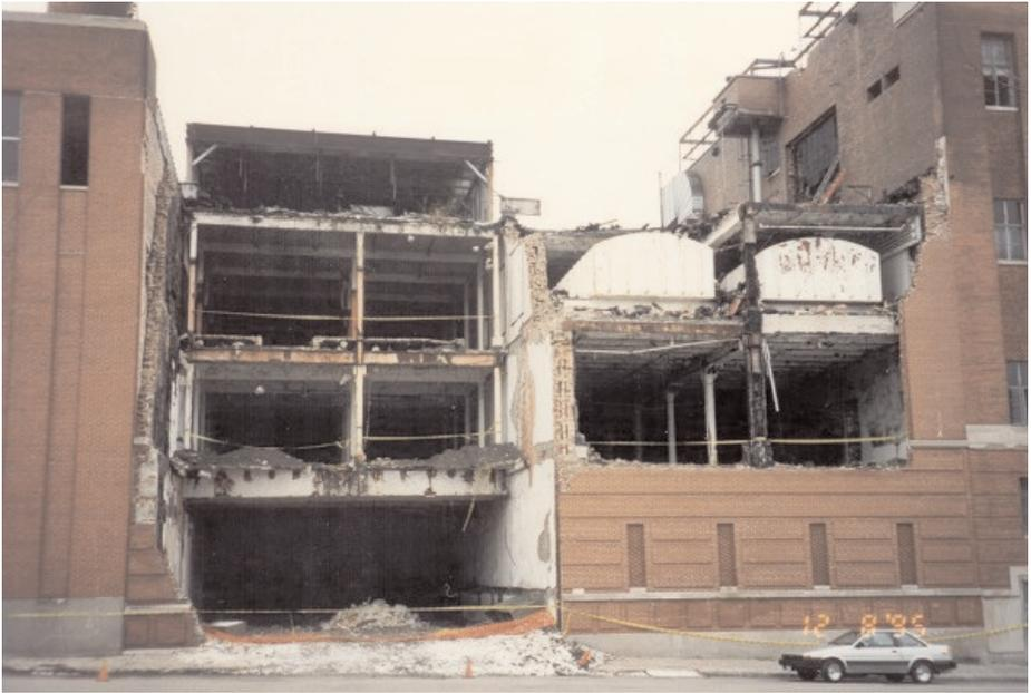
*Figure 19. The northeast side of the Hudepohl brewery complex, as it appeared after a fire inside the abandoned facility in September 1995. (author's collection)*
