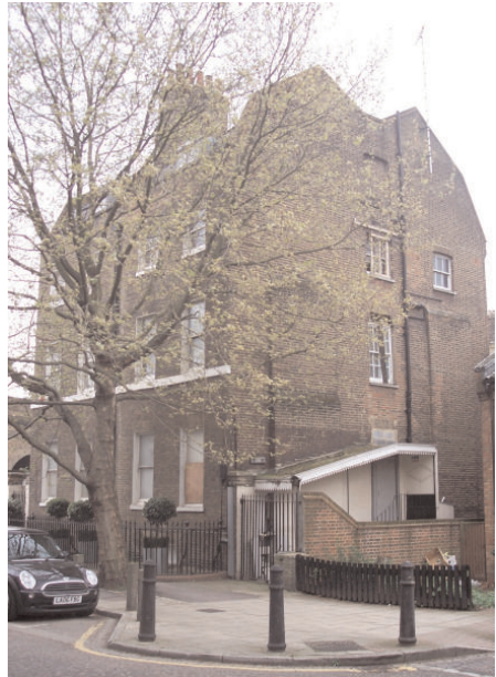
Figure 2. 21 and 23, Park Street, Southwark, built in about 1820 for senior employees of the Anchor Brewery (then owned by Barclay & Perkins Co., and later by Courage). Charles Spurrell and his family lived at No. 23 from about 1820 to 1835.
