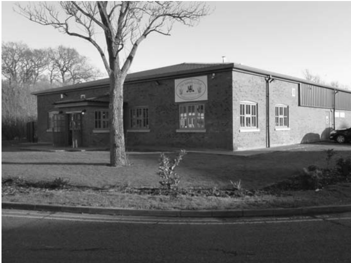
Figure 5. An exterior shot of Belvoir Brewery.
