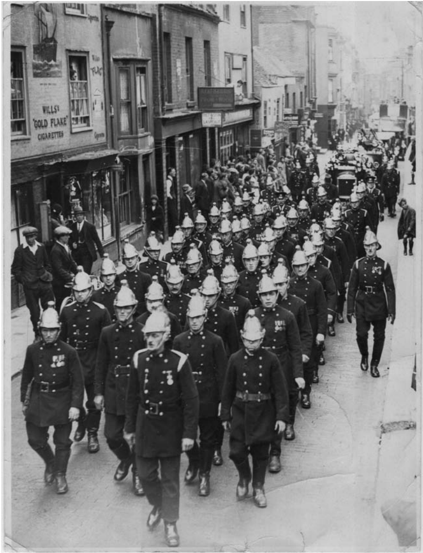
Figure 2. The FILO in the 1920s with the fire brigade's march taking place
