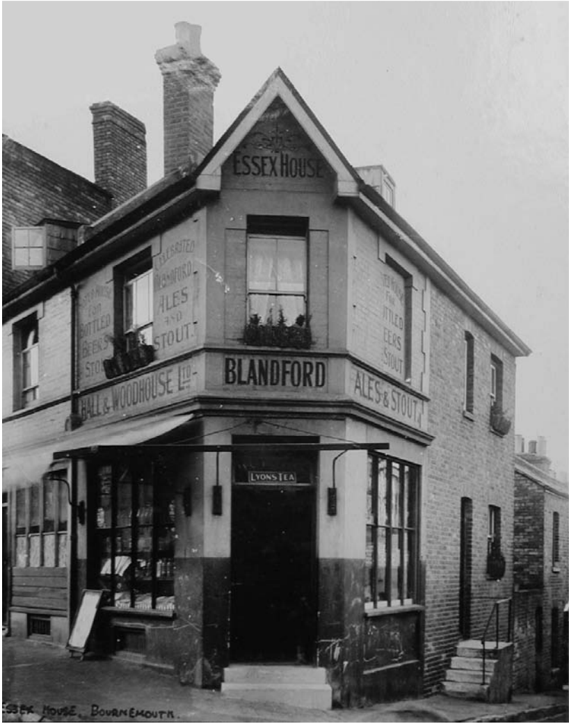
Figure 7. Essex House, Bournemouth.
