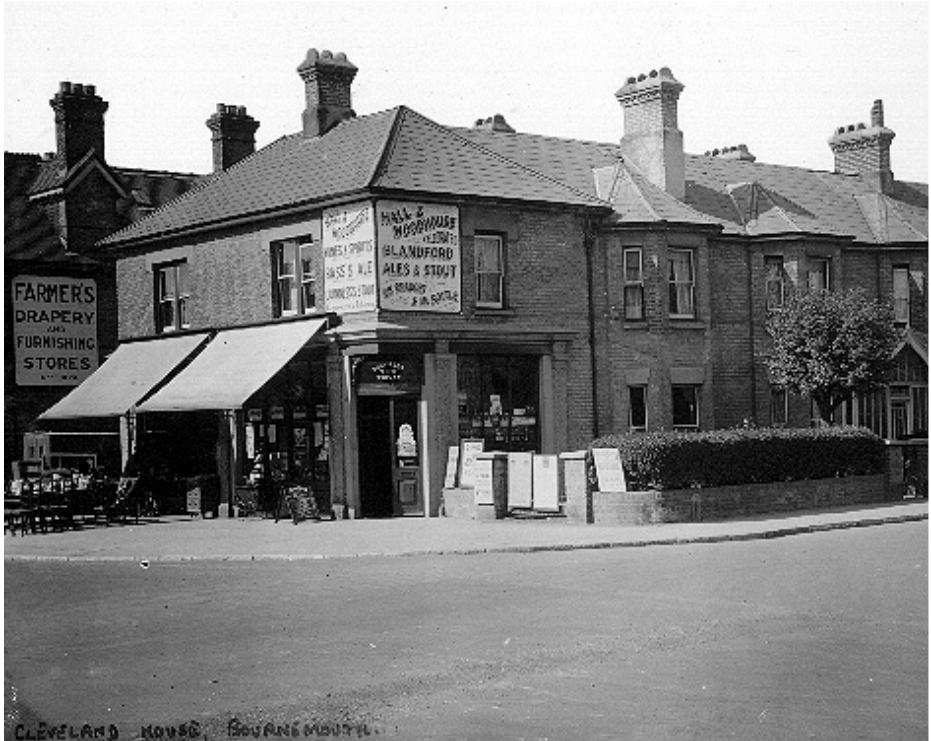
Figure 8. Cleveland House, Windham Road, Bournemouth.
