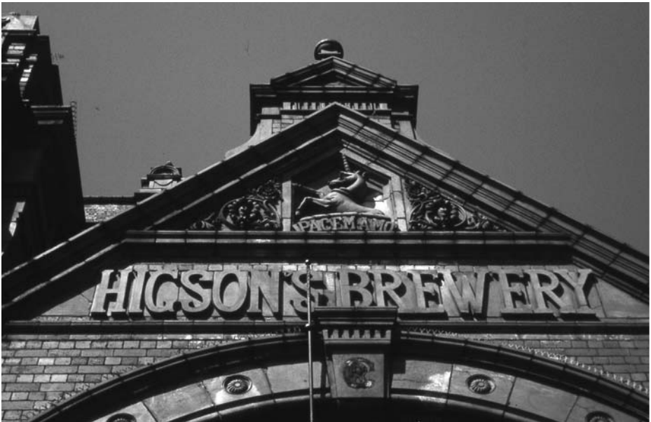
Figure 3. Terracotta work on the Mersey Brewery reflecting its sale to Higson's in 1923.
