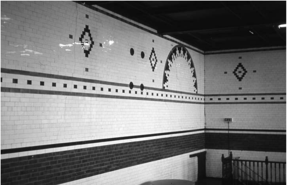
Figure 1. Decorative glazed brickwork in the former hop store of the Mersey Brewery, Liverpool.
