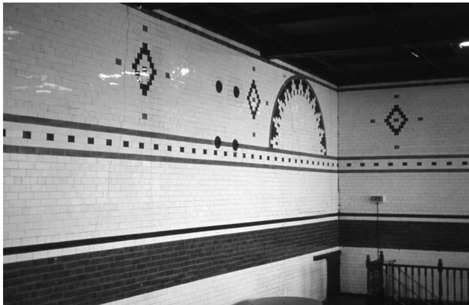
Figure 1. Decorative glazed brickwork in the former hop store of the Mersey Brewery, Liverpool.
