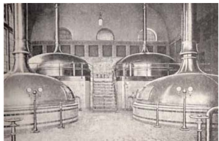
Figure 15. The brewhouse of the Hanover Brewery Company c. 1900 showing left to right, the mash copper, the mash tun, the lauter tun and the wort copper.
