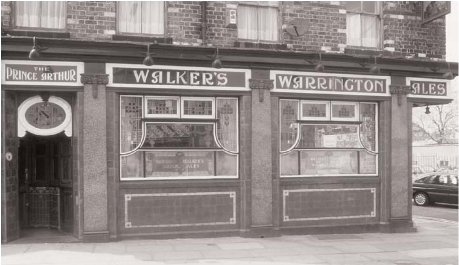
Figure 19. The Prince Arthur, Walton, Liverpool, has a distinctive Taylor Walker tiled frontage of c. 1905. The windows have etched glass to create the sense of separation between the pub and the outside world.
