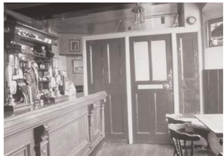
Figure 7. A simple screen such as that at the Nova Scotia in Bristol Docks where it divides the small private bar from the public bar was a cheap and easy way of creating multiple spaces in Victorian pubs.
