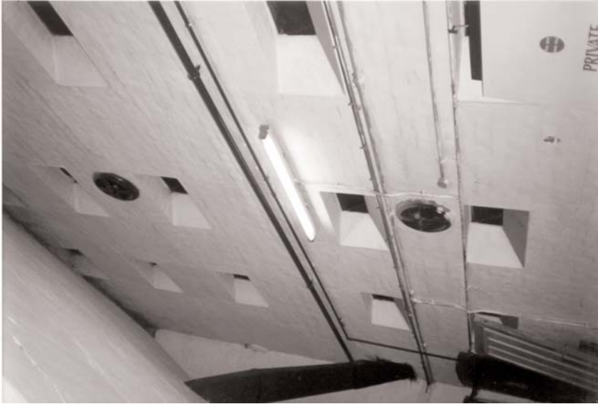
Figure 11. Malthouse No 4, Weymouth - Last's patent ventilator - interior.
