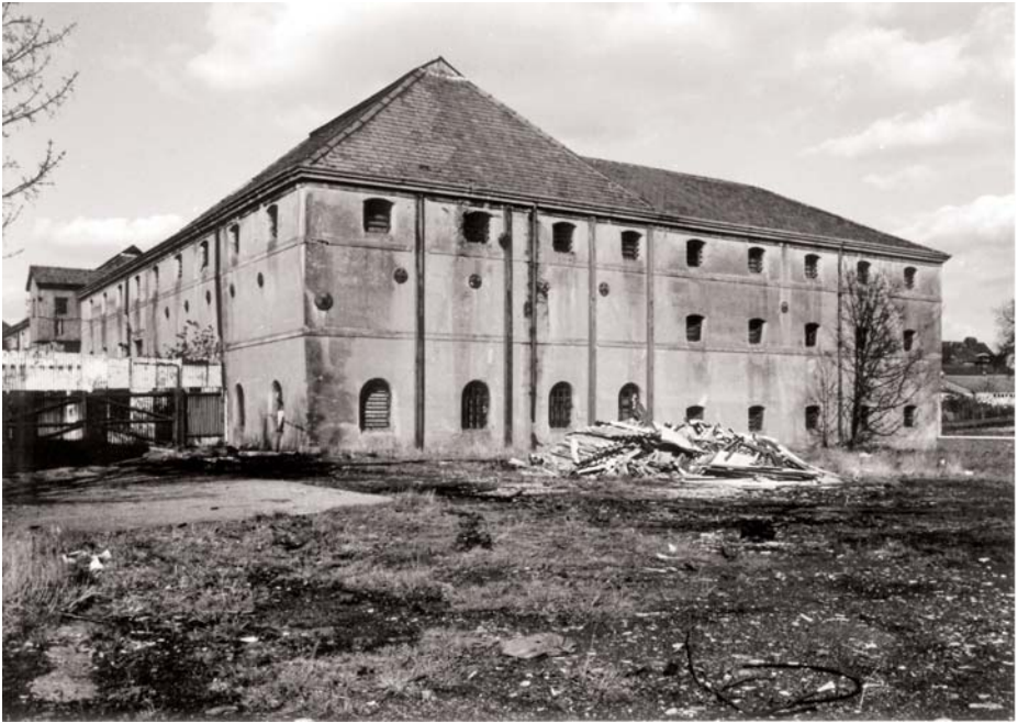
Figure 1. South block of the mass concrete maltings, Trentside, Newark-on-Trent, Nottinghamshire
