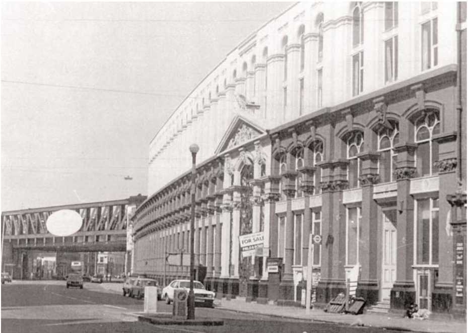
Figure 5. Hop Exchange, Southwark Street, 1983.
