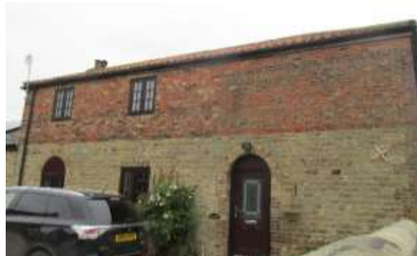
Low Street Hop House
