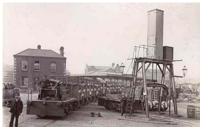
The hydraulic lift used to lower a narrow gauge loco into the bogie
