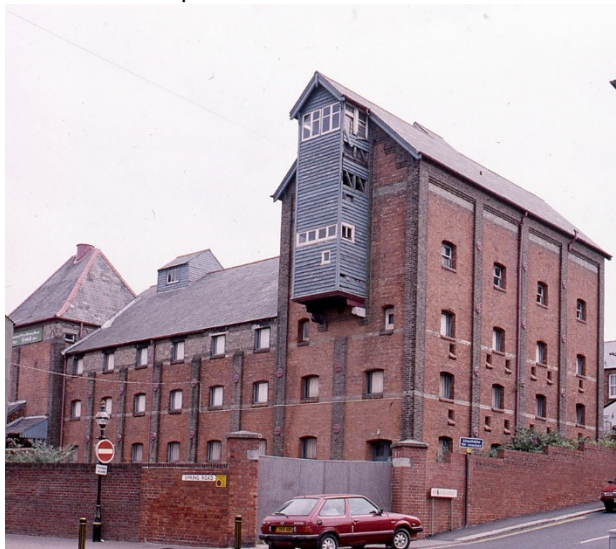
Groves Malthouse No4 in Weymouth showing the ventilators between the windows in the old barley storage/steeping block.
