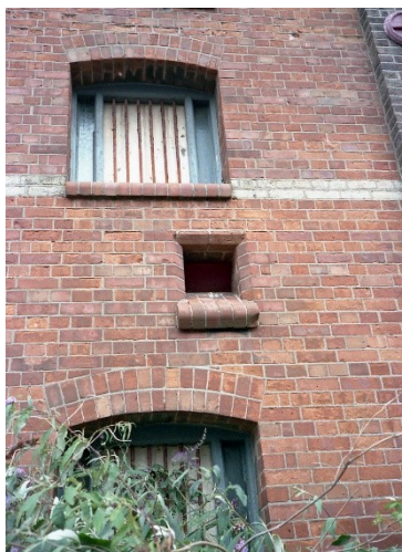
Detail of the ventilator orifices
