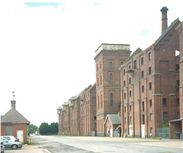
One of the fire damaged east malthouses
