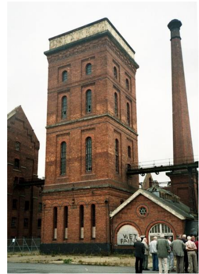
Water tower and chimney stack
