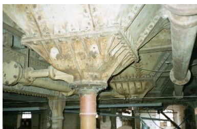
Extant internal features; from top left: Germination floor; odd pulley; spiral stairway to water tower; base of the steep tanks, massive support girders and the mechanism to open the kiln louvres
