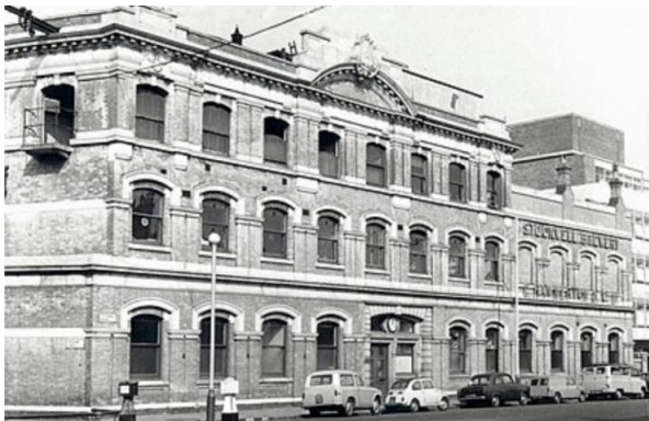
Stockwell Brewery frontage shortly before demolition in 1965.
