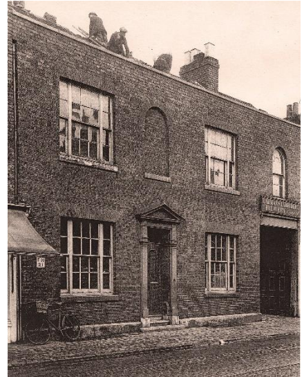
Demolition in progress
